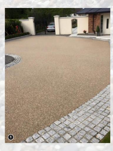
Factors effecting choice are: colour, hardness, texture. Pathways can use all but the softest aggregates: drives will require pea gravels, granites or basalts which are more durable. Steep drives will require an angular aggregate to ensure good grip, whilst a drive likely to have children playing around, may require a rounded pea gravel.
